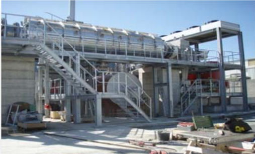
New construction fro CBp – Tyre scrap pyrolysis plant [Cyprus]
