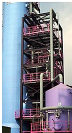
New build gas scrubber blast furnace 8
