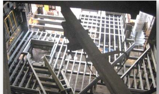
HO 3 Relining for Arcelor Mittal Bremen
